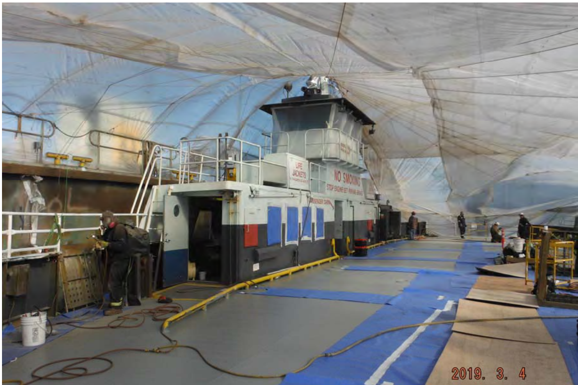
Photo No. 8 Main deck looking aft from No. 1 end
