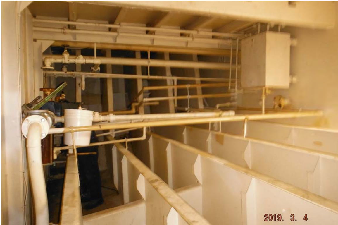
Photo No. 7 Interior void, representative sample of internal coatings
